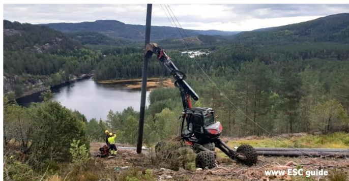
MENZI MUCK #Construction of #HighVoltagePoles
