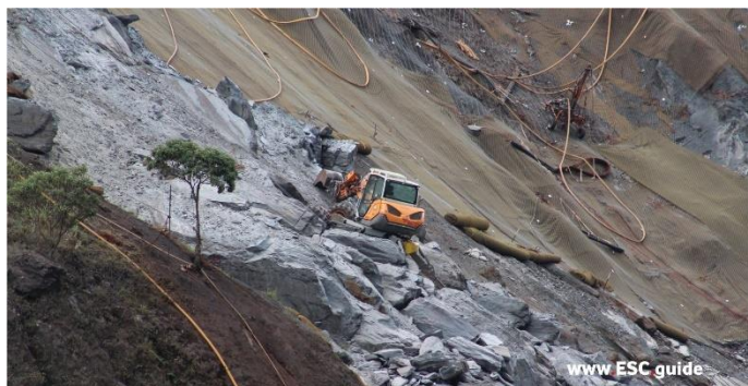
MENZI MUCK #LandslideRepair
